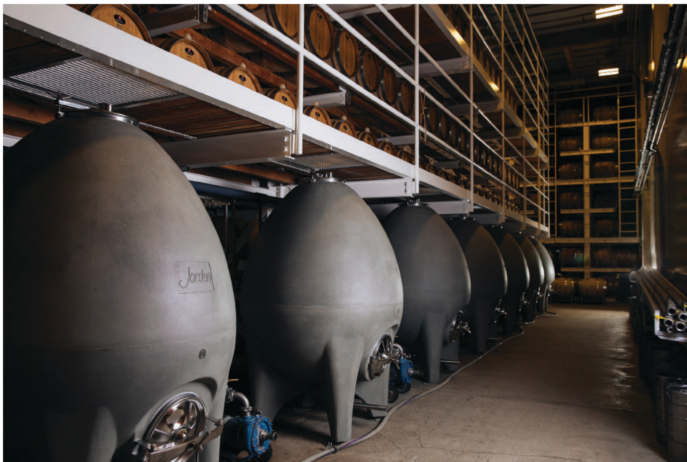
The Jordan cellar houses eight concrete eggs.
